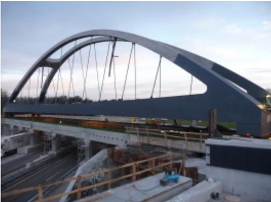
The insertion of the second structure, a railroad bridge weighing 300 tonnes with a length of 80 meters above the motorway in St.Margrethen, was a much more complex operation. This bridge was first displaced longitudinally by 70 meters after its construction, then moved 20 meters laterally, lowered by 3.5 meters and finally tilted through 80 cm on one side in the longitudinal direction.
